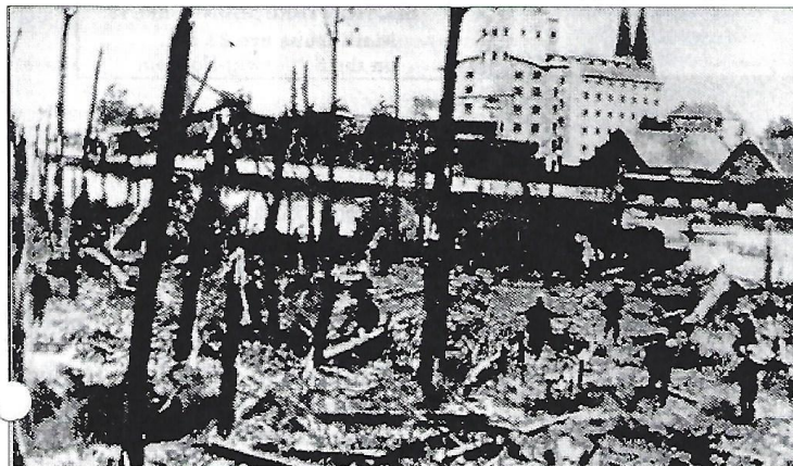
German troops penetrating the Westerplatte following the capitulation in September 1939. Neufahrwasser is in background. Some buildings were flattened by the concussion of the S-H's 23 cm big guns.
